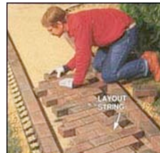
LAY THE PAVERS using a string guideline. Cut and install pieces that build up to the border later.
