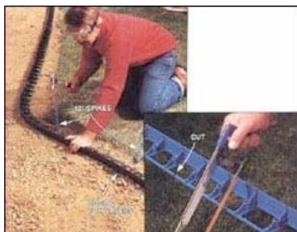
6. INSTALL THE SNAP EDGE on the tamped subbase using 8" - 10" spikes. Cut the webbing on the edging's back side to make it flex for curves
