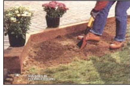
16. LANDSCAPE around the complete patio with flowers, shrubs and grass. Grass will root through the open spaces in flexible edging to anchor it in place.
