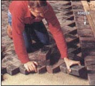
9. INSTALL THE PAVERS starting along the longest, straightest edge. Border pavers provide a crisp finished edge, especially along curved portions of patio.
