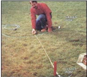
1. OUTLINE the patio perimeter using a garden hose for curved areas and long 2x4s for straight sections.
