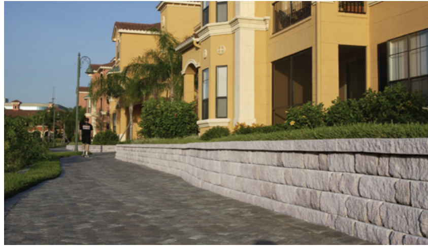
Each parking lot was separated from the landscape by a retaining wall that defined the grade.
