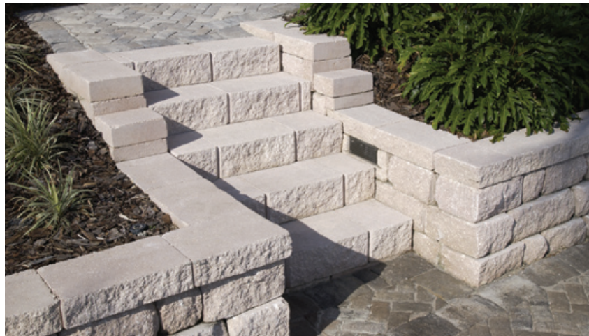
Light units were installed for safety on steps constructed with the Highland Stone® retaining wall system.
