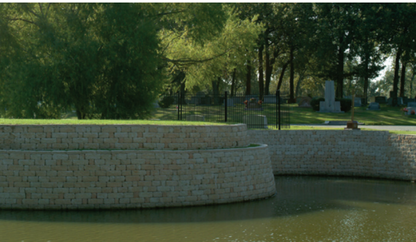
The blended color of the rough, rock-like texture of the multipiece system helped the product fit with the rustic granite shore walls that remained in place.
